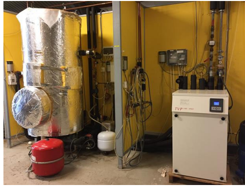
c) Combi-storage and heat pump
