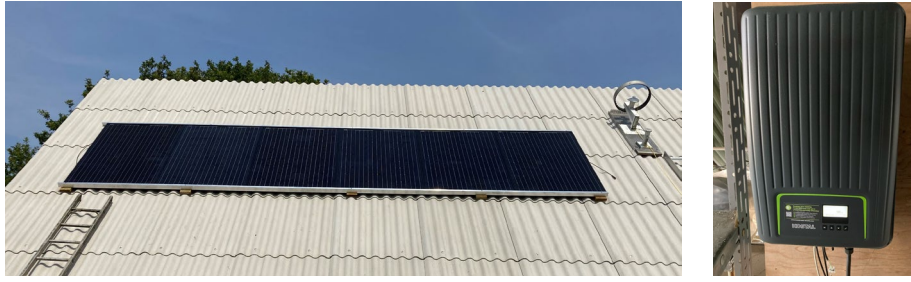
Fig. 3: PV panels on the roof of the test facility (left) and the inverter (right)
