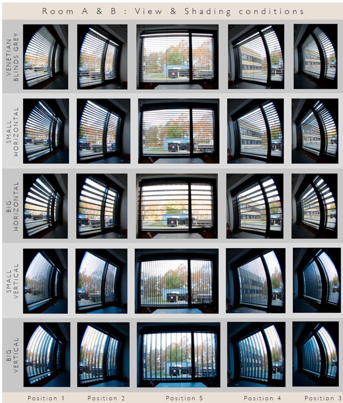
Fig. 4. Cropped Fisheye images from each position showing the each window view condition through different solar shading.
