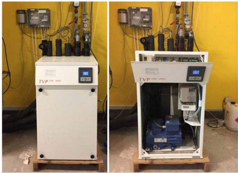
Figure 1.6: Heat pump (heating capacity of 3-12 kW).
