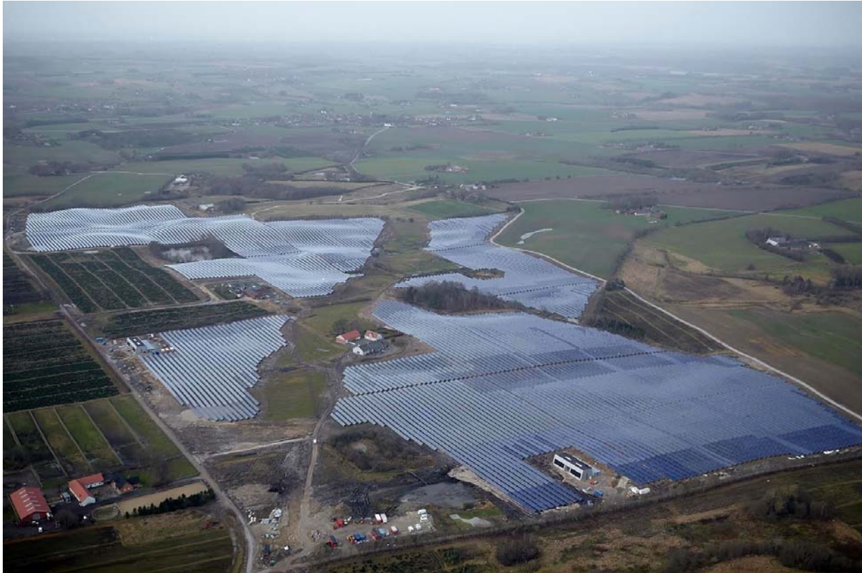
Fig. 10: Solar heating plant in Silkeborg, Denmark [11]
