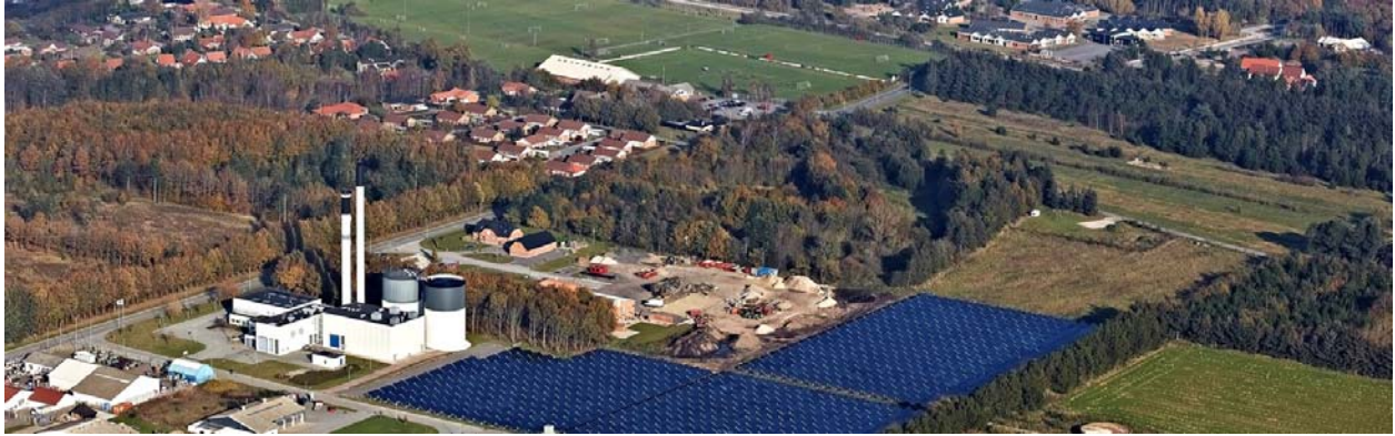
Fig. 11: Aerial view of Sæby solar heating plant
