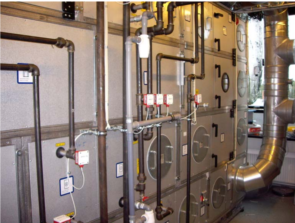
Figure 2. The ventilation system for the test room that can supply air simulating different outdoor climate conditions.
