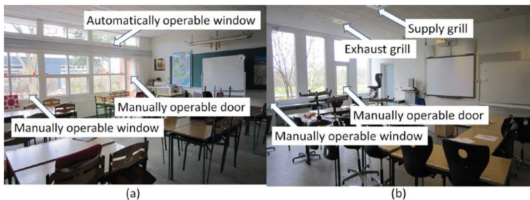
Fig.2 The classrooms in Wings A & B and the main building
