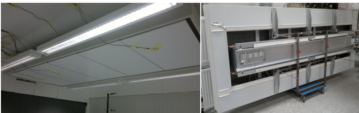
Figure 3.10: Chilled beam with radiant panels made by Halton.
