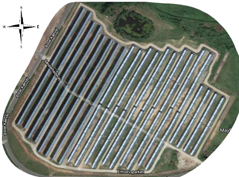
Figure 4.1: Parabolic trough collector solar field in Brønderslev. [11]
