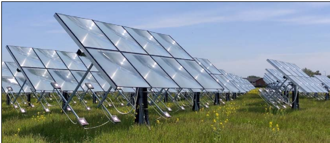
Fig.11. Photo of the Fresnel lens solar collector field, Lendemarke, Denmark.
